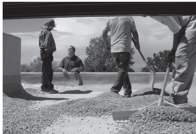
Figure 3. Some roofers protect SPF roofing from ultraviolet light with crushed stone ballast. Stone ballast only works on relatively flat roofs. [Photo credit: Thermal Coatings and Insulation]
