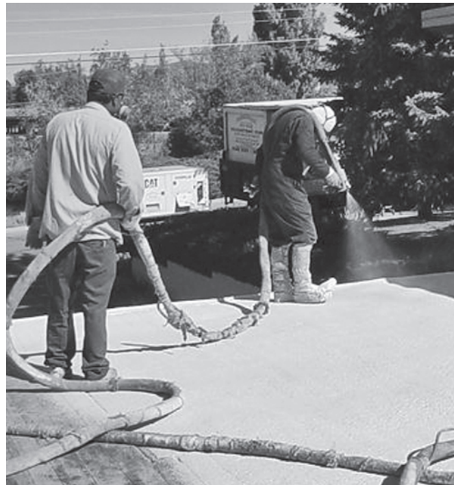
Figure 2. Spray polyurethane foam roofing can only be installed when the weather is warm, dry, and relatively windless. [Photo credit: Goodrich Roofing Co.]
