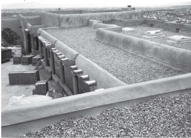
Figure 1. In the Southwest, where traditional architectural styles favor flat roofs, spray polyurethane foam roofing is fairly common. The SPF roofing on this home is covered with aggregate ballast. [Photo credit: North Carolina Foam Industries]
